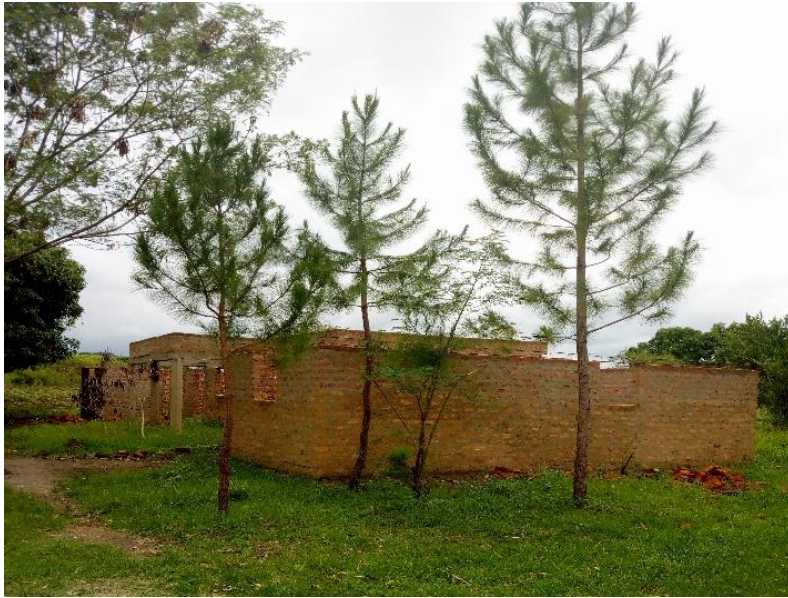
Parish House under construction 1
