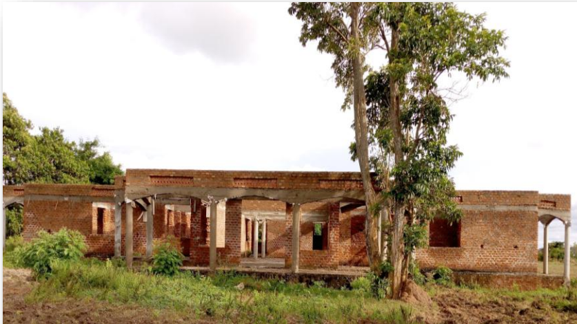
New Parish House under construction
